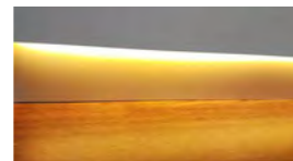
Installation plinthe / Skirting light installation
